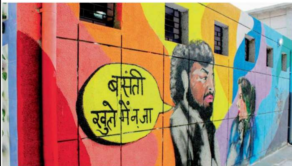
A renovated toilet in Sultanpuri.
